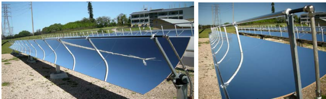
NEP Solar Pty Ltd. collector PolyTrough 1200 with MIRO-SUN®
